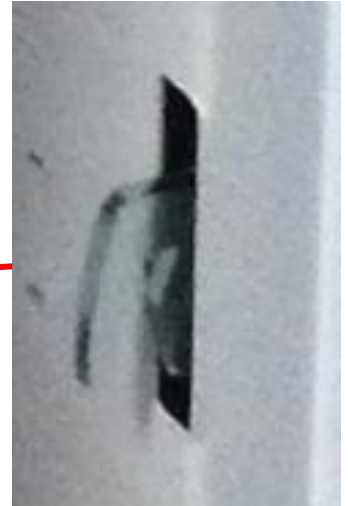
Detail of lock cam when locked condition
